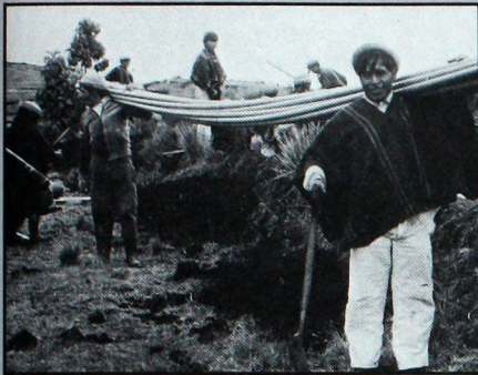
Community members in Palugsha install pipe to bring well-water to homes. The women dig, and the men carry and install the pipes.
